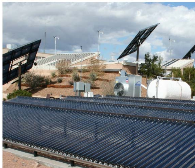
FIGURE 2: DEMA SOLAR COOLING SYSTEM
