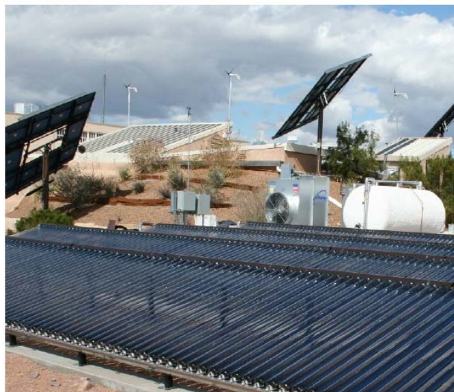
FIGURE 2: DEMA SOLAR COOLING SYSTEM
